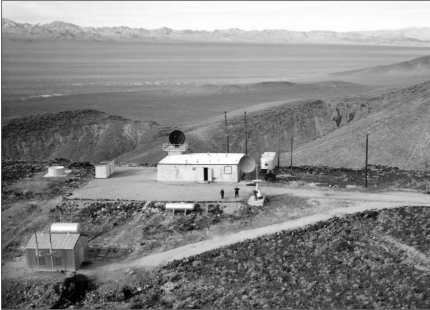
The High Range stations were positioned on top of mountains to provide the best look angles for the radar and telemetry receivers. The Beatty, Nevada station was closed when the X-15 program ended and nothing remains at the site except for the concrete slabs where the buildings once stood. (NASA)
