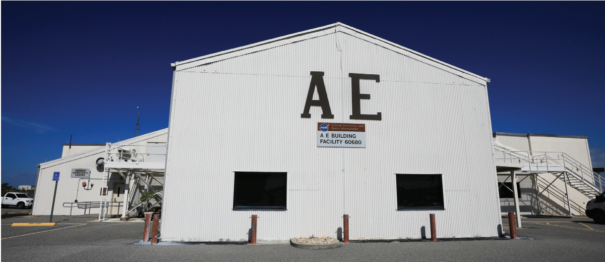
Hangar AE at Cape Canaveral Space Force Station in Florida houses control rooms providing real-time voice, data, and video information for expendable launch vehicle checkout and operations, and is used to support the uncrewed launch vehicle fleet. Photo credit: NASA/Ben Smegelsky
